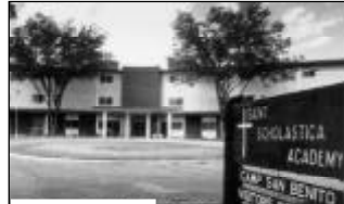
St. Scholastica's entrance and one of the original brick buildings which is still in use today. The Benedictine Sisters founded this all girls boarding and day school at 6th and Pike in Cañon City which they operated for 111 years.
